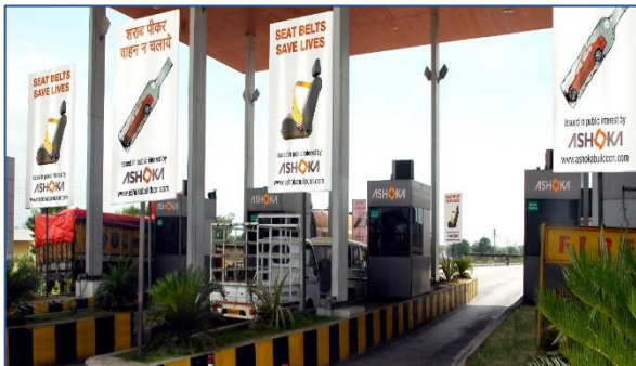
The Durg Bypass Project
