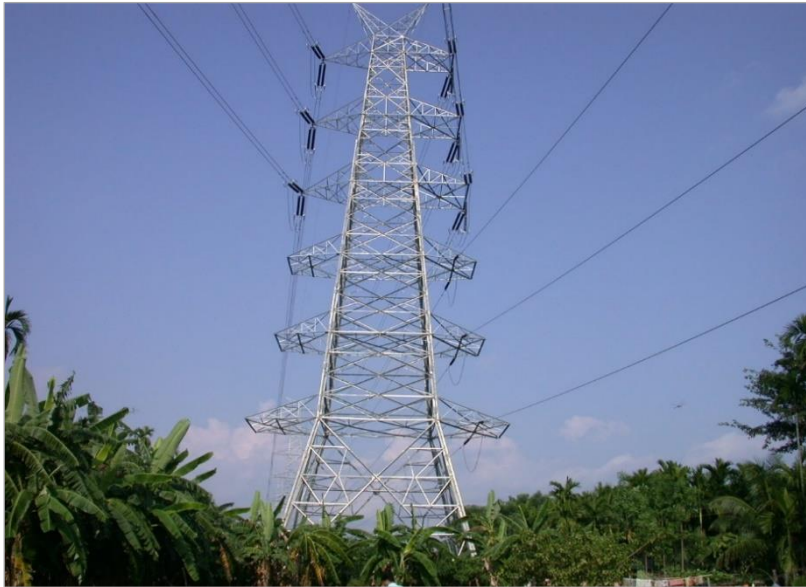
Figure 1: Multi circuit towers conserving Right of Way: Eco –friendly outlook 1
